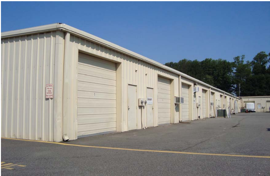
REAR WORKING COURT OF COMPLEX
