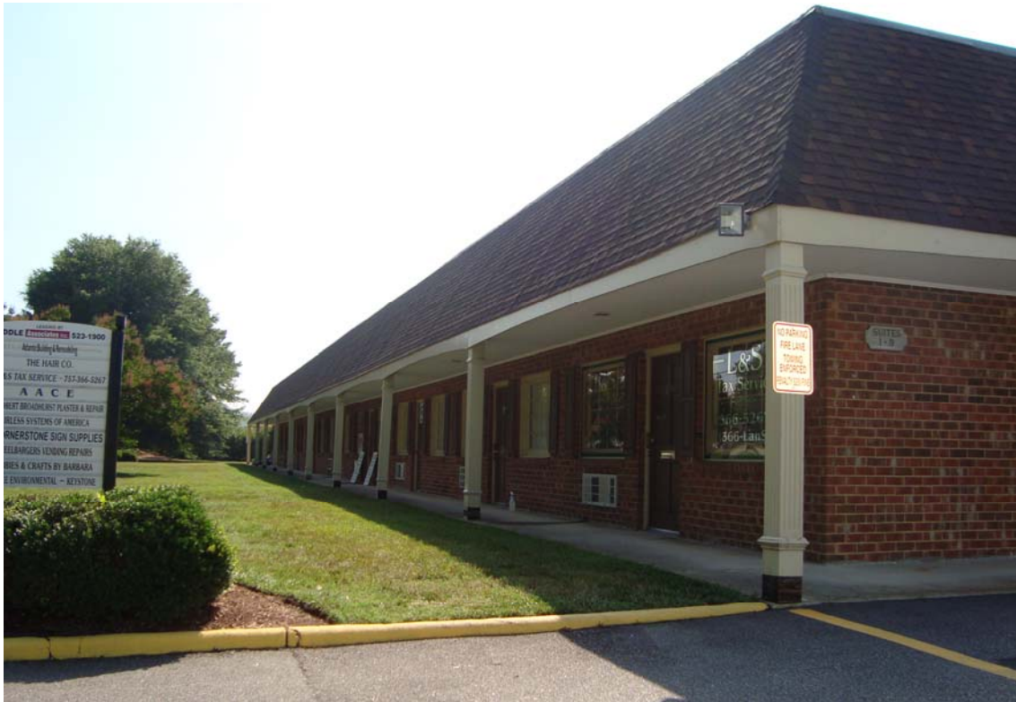
STREET FRONT OF COMPLEX
