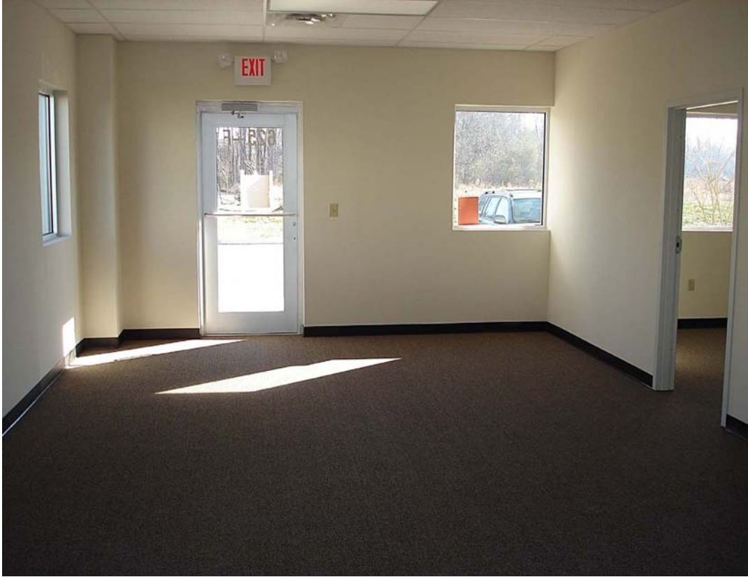
Unit F Office Build Out
